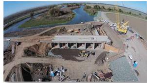
Reclamation District No. 108 began construction on the Wallace Weir Fish Rescue Facility Project in August 2016. The \$13.3M project involves constructing a permanent weir with a positive fish barrier and fish collection facility. The fish collection facility would be adjacent to the fish barrier and work in tandem with the
